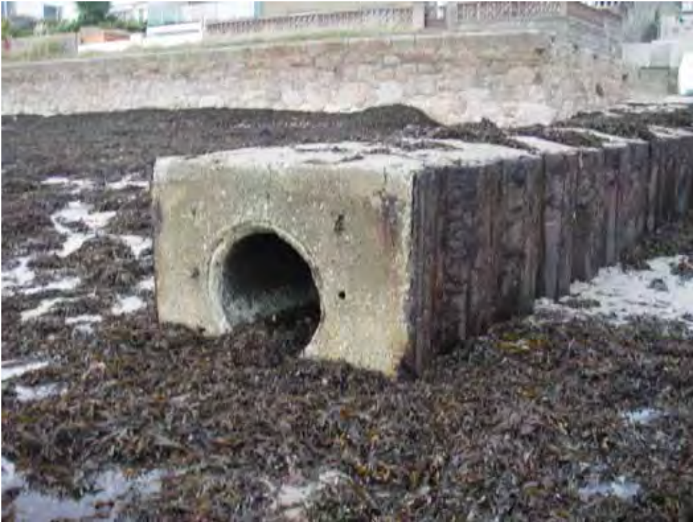
Figure 6. Outfall at La Commune de Pontac
