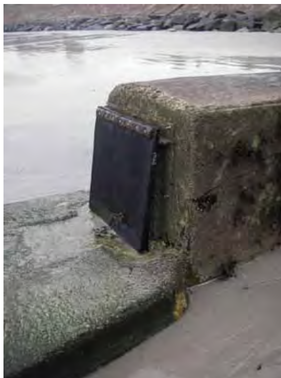
Figure 15. Outfall with flap valve north of Round Tower No. 5
