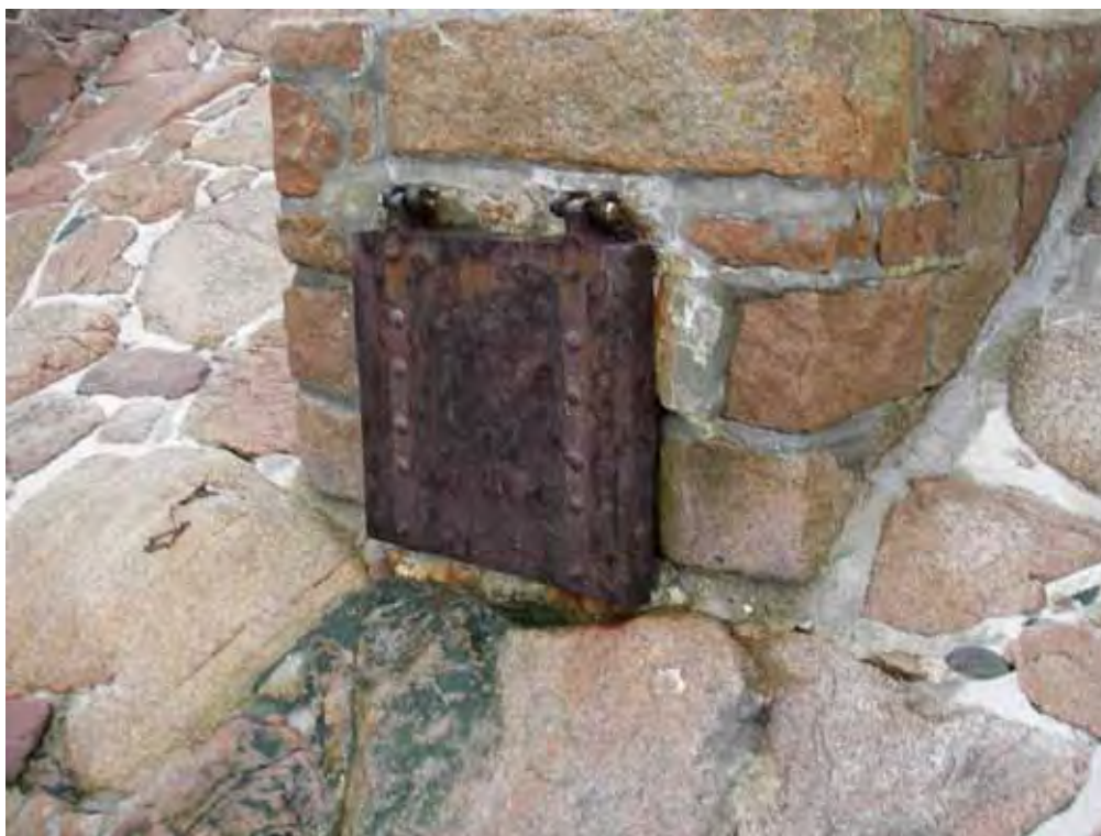
Figure 8. Flap valve at Pontac slip
