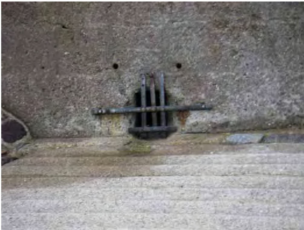
Figure 19. Drain outlet in sea wall south of Round Tower No. 2
