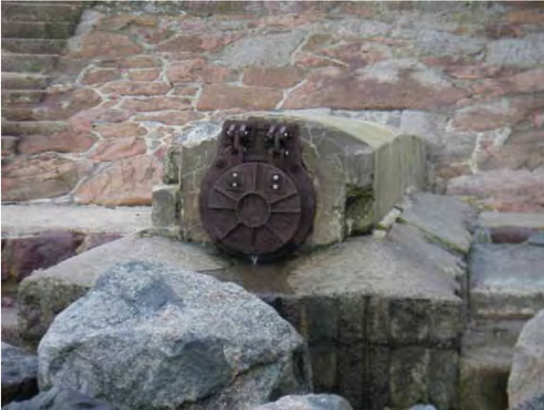
Figure 18. Flap valve in sea wall north of Round Tower No. 2
