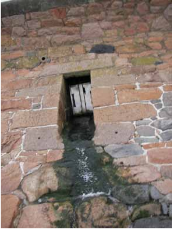
Figure 7. Culverted flow through sea wall near Pontac slip
