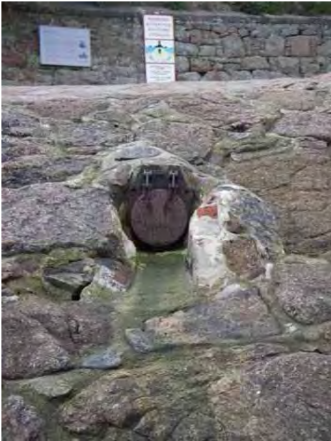
Figure 20. Flap valve in sea wall north of La Nez de la Rocque
